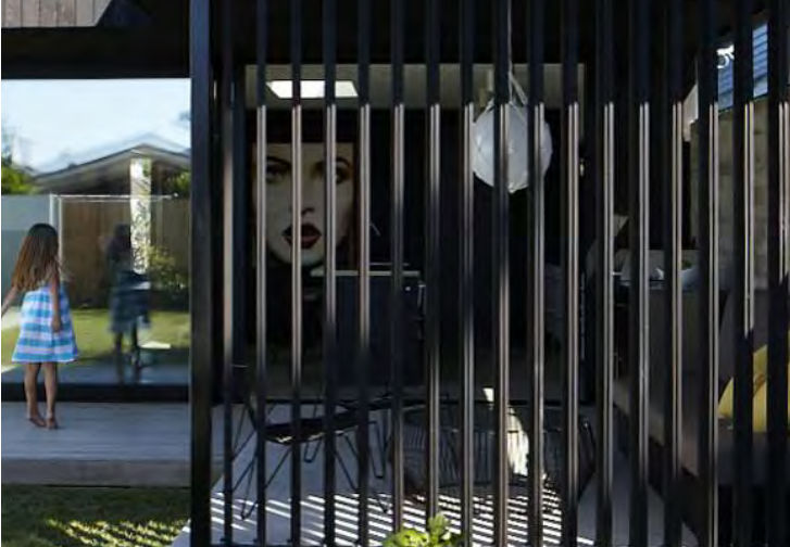
SCR-01 VERTICAL LOUVRED MAIN ENTRY SCREEN, POWDERCOATED FINISH SIM/EQ TO DULUX 'WOODLAND GREY'
