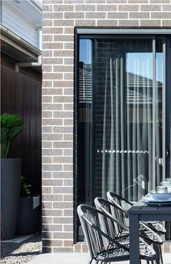
FBK-02 SIM/EQ TO AUSTRAL BRICKS WILDERNESS DESIGN 'BLACKBUTT', BRICK PATTERN : STRETCHER BOND
