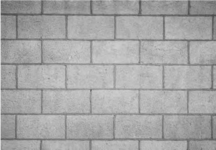
BLK-01 CONCRETE BLOCKWORK. PATTERN : STRETCHER BOND
